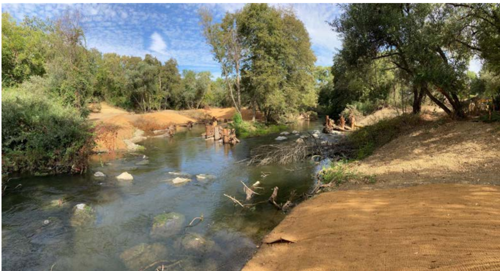
Photo shows view looking upstream at newly installed mainstem boulder fields. Outlet of river right side channel (Stromberg property) visible in middle-left of photo. Wood structures at inlet to the side channel on river left (Gros-Balthazard property) visible in middle-right of photo. Photo taken September 8, 2021.
