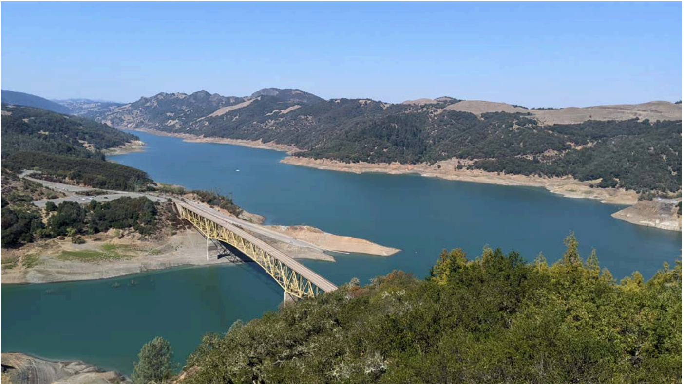
Lake Sonoma, September 24, 2021 when the reservoir was approximately 45% of capacity with 110,600 acre feet of water in storage.
